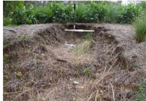
Irrigation Blowout
